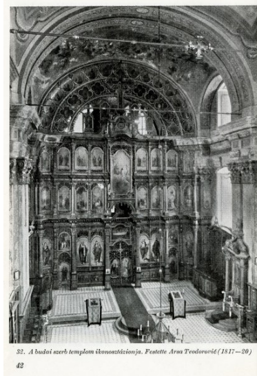
Figure 1: The view of the iconostasis in its original appearance before demolition of the church
